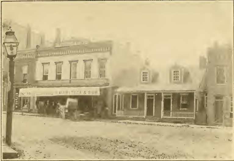
Switzer Building Waterman House [Pages 192, 354]
